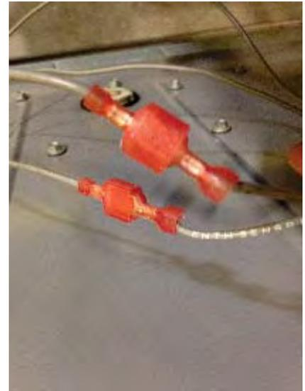
DISCONNECT TWO GREY WIRES IN FILTER SECTION OF THE RTU. THESE WIRES ARE LOCATED IN THE FACTORY WIRING BUNDLE ("PL-6"). ONE IS LABELED ENTH SENSR"AND THE OTHER IS UNLABELED. ONCE REMOVED CONNECT FEMALE ENDS TO R/A SENSOR AS SHOWN ABOVE
